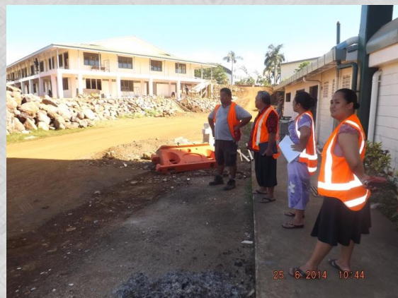
LTD Team on Site with Lucky Construction Team Leader
