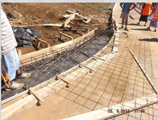
Footpath Construction Work
