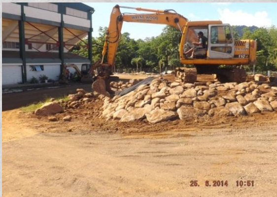
Landscaping works by Lucky Construction
